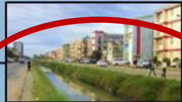
Urban drainage phase 1 – World Bank
