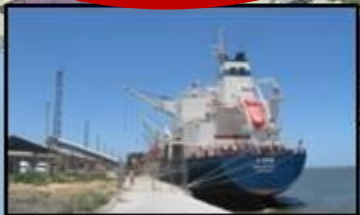
Expansion of quays – CFM/Cornelder
